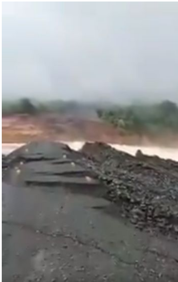
Fig. 6 - https://twitter.com/Zeno7Inc/status/1021680781498888192 video showing the section of the dam that was broken, with the water flowing below.
