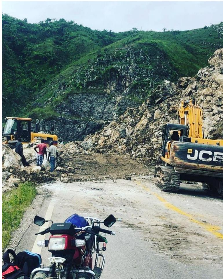
Fig. 3 – Haitian Civil Protection clearing the landslide that blocked RN#7 (source: Civil Protection facebook page).
